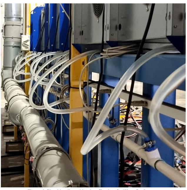
Figure 1. Plumbing line with take off points for WaterGenius
